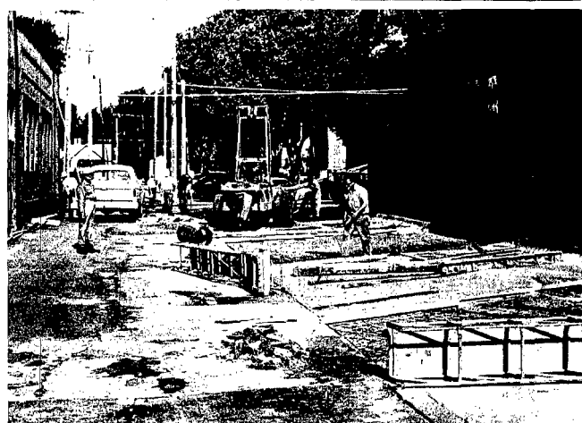
THE SAND PILE is gone. Where once only loose sand lay south of the Wayne Herald building, now there is concrete paving. By the time this picture is published, all the area around the building will be paved to provide additional off-street parking. The paving crew is shown here as they prepared to start pouring Monday morning. Side-walk superintendent overseeing the job is Skilor Bill.
